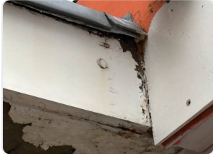
Afbladderende betonluifel
